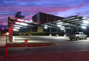
Photovoltaic Installation for SunPower at the Porterville USD
